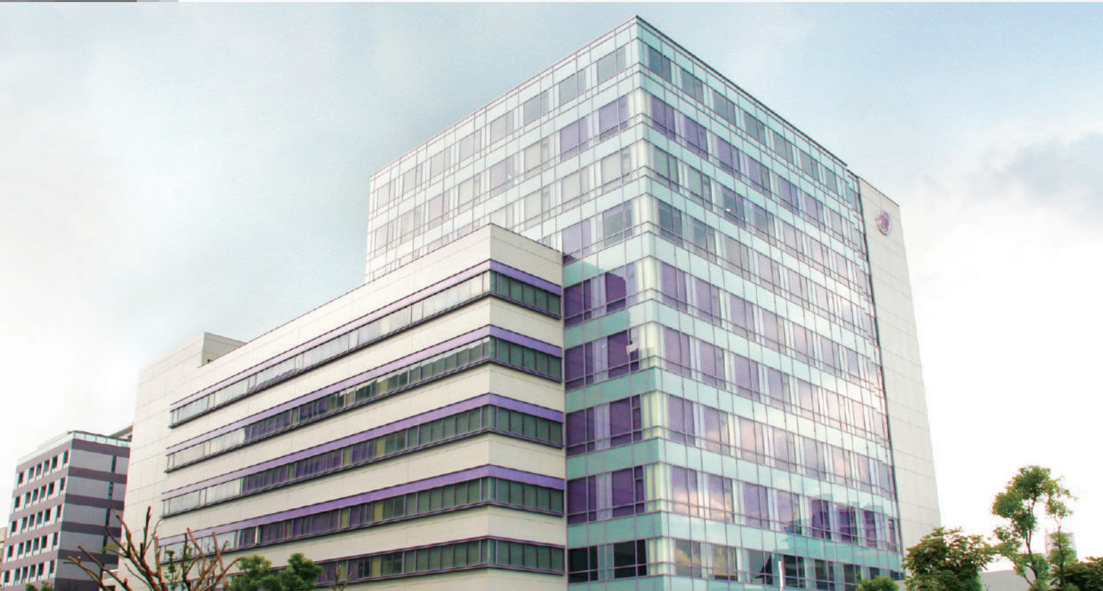
Portwell Engine (PE) Building
